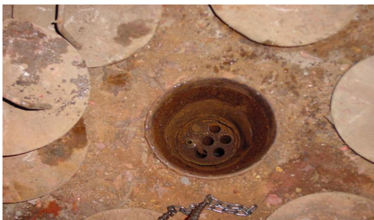
Fig. 13.1. Can made of carbon steel, without a protective plug, with two SFA
