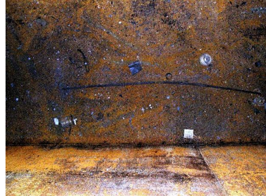
Fig. 13.13. Right large pool, photo-fragment with plugs from multiple-use canisters at the bottom.
