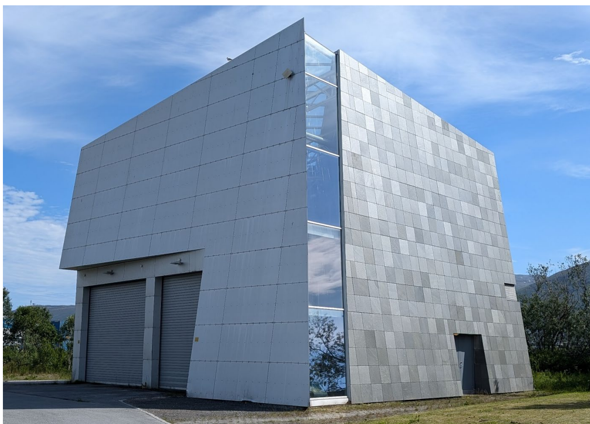
Figure 4. The Breivika wastewater treatment plant (Photo DSA).
