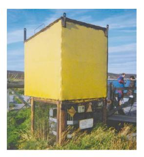
A RTG with the enclosure and power supply. Photo: The Norwegian Radiation Protection Authority
