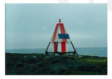
An alternative to RTGs: A lighthouse fitted with a solar panel that generates electricity. Photo: Office of the County Governor of Finnmark
