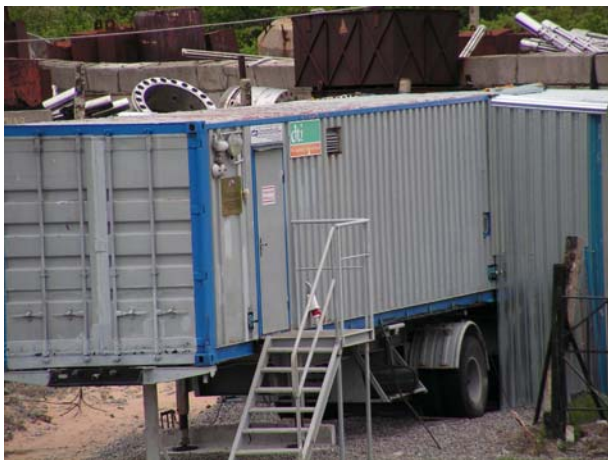
Mobile decontamination facility (sanitary pass/check point) on the industrial site SevRAO facility no. 1 at Andreeva Bay.
