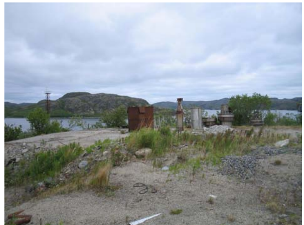
SevRAO facility nr 2 at Gremikha – view of the radioactive waste and SNF
