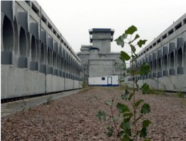
Figure 5.7 – ChNPP dry interim spent fuel storage facility
