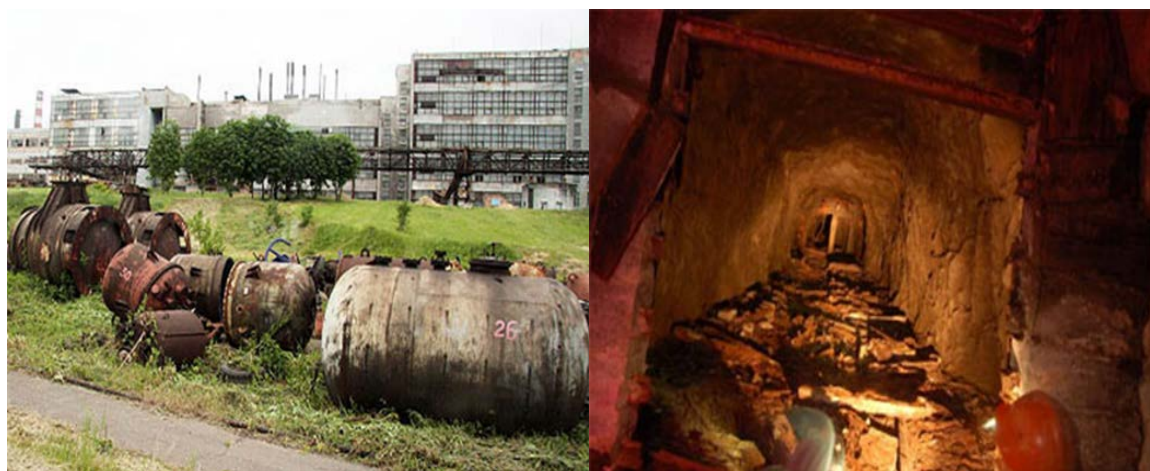
Figure 6.2 – Abandoned PChP objects negatively affecting people and the environment
