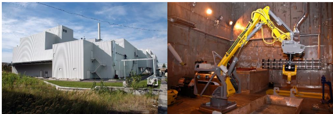
Figure 5.3 – Chernobyl NPP solid radioactive waste treatment plant (SRTP)
