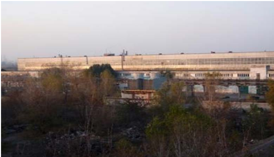
Figure 6.1- Part of Prydniprovsk Chemical Plant territory
