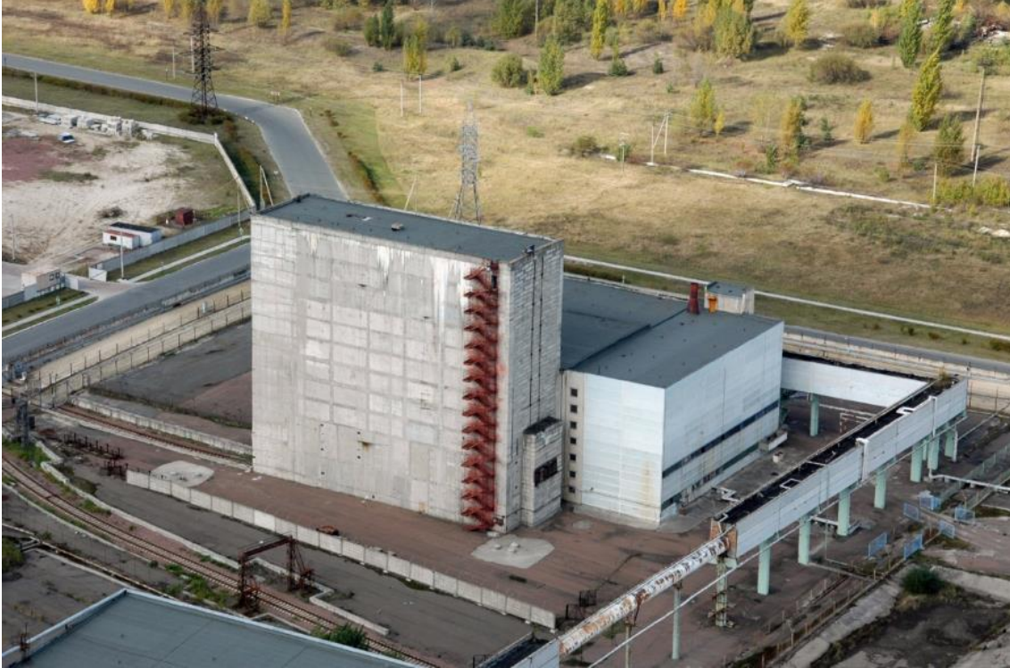
Figure 5.5 – ChNPP wet interim spent fuel storage facility
