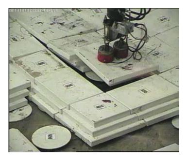
Figure 3. Installation of the biological shielding on the surface of the DSU-3A tank.
