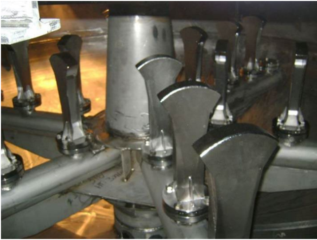
Fig. 3.2 – Venturi nozzles used in a scrubber for high-rate filtration of steam-gas mixture
