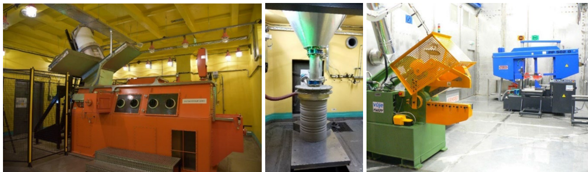
Fig. 6.3 – SRTP ZNPP incineration and fragmentation facilities
