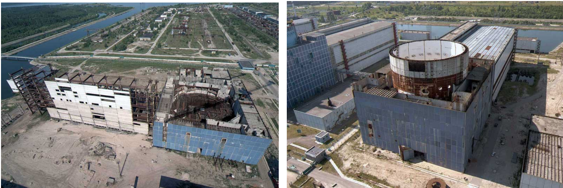
Fig. 3.7 – Construction status of KhNPP Units 3 and 4
