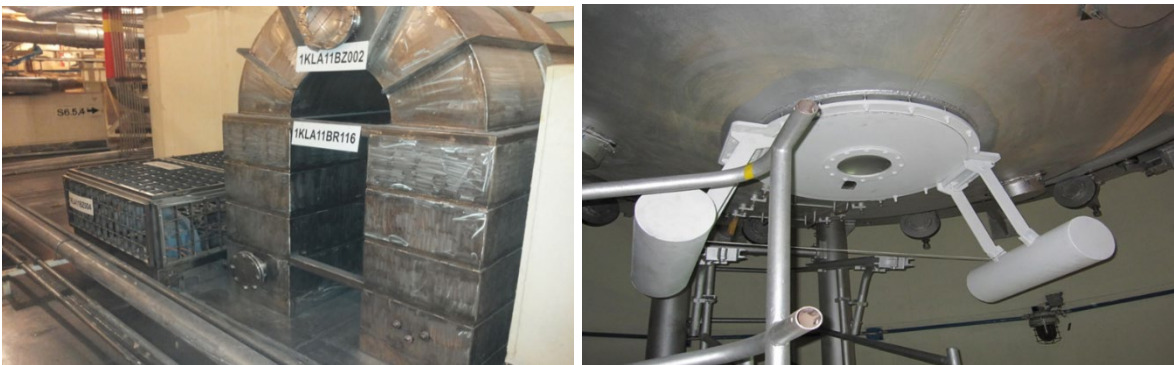
Fig. 3.3 – Equipment for the ex-vessel reactor cooling system (hydraulic seal of the ex-vessel reactor cooling system and floating mechanism to open the hatch of the protective screen of the reactor pressure vessel)
