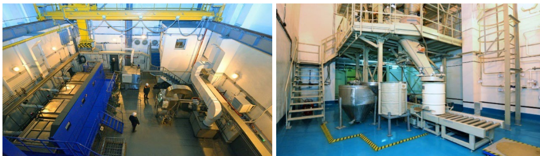
Fig. 6.2 – SRTP RNPP metal decontamination and cementation facilities
