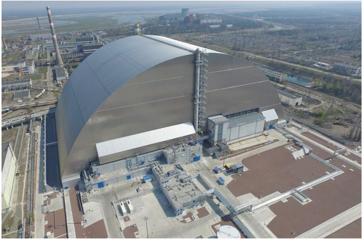
Fig. 6.8 – New Safe Confinement
